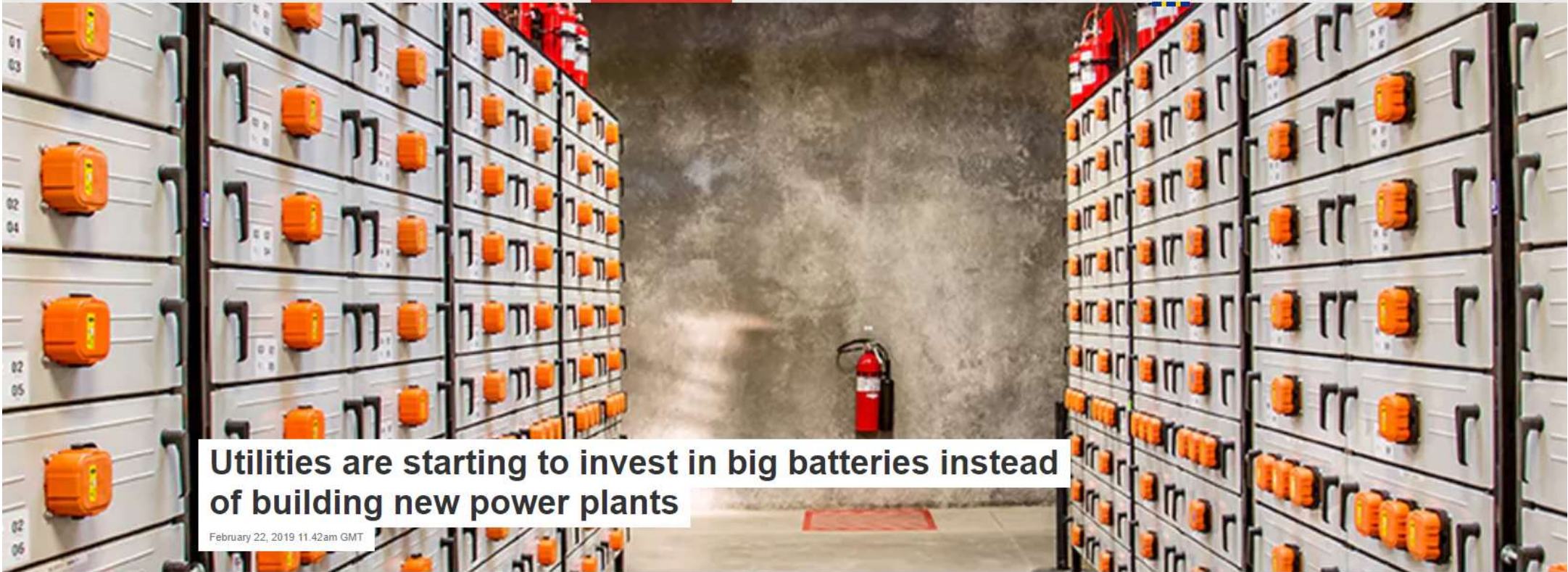
This is what a 5-megawatt, lithium-ion energy storage system looks like. Pacific Northwest National Laboratory
